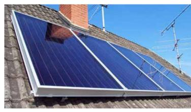
It is common to position and fix collectors above roof tiles. Alternatively, some systems can be integrated into the roof for a less intrusive finish. Your OFTEC registered solar thermal installer will be able to discuss which type of collector and mounting option best suits your needs.
